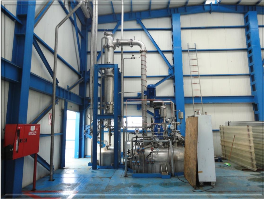
Reactor assembling and piping
